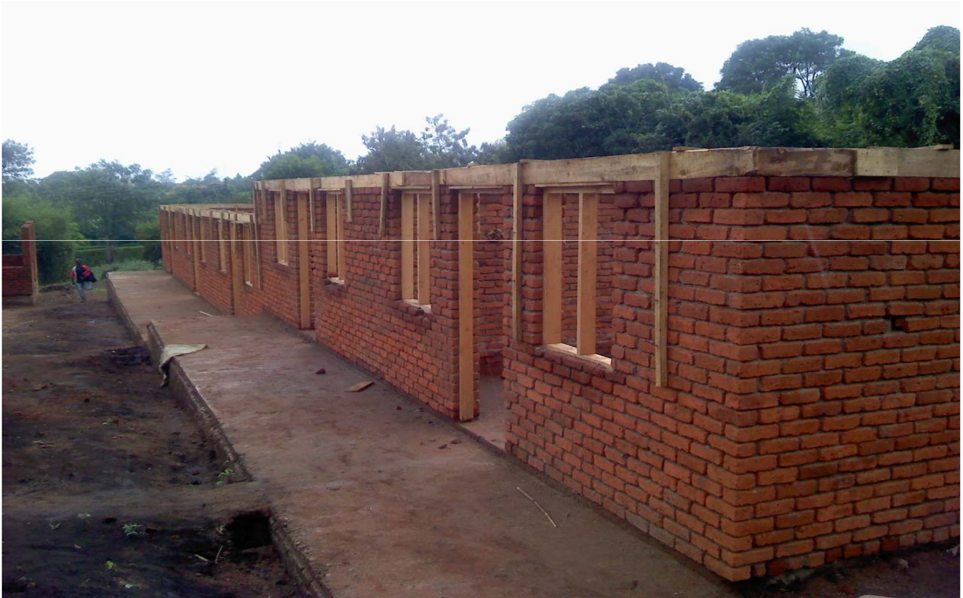
Pic. 5: Women shelter; Front view, about to complete ring beam
