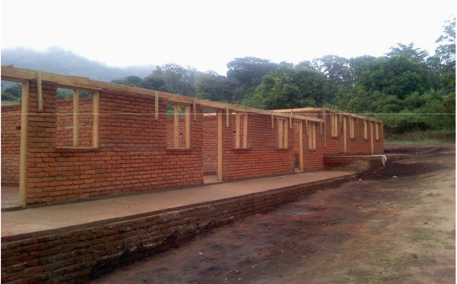
Pic. 4: Women's Shelter; Front view, about to fill ring beam concrete
