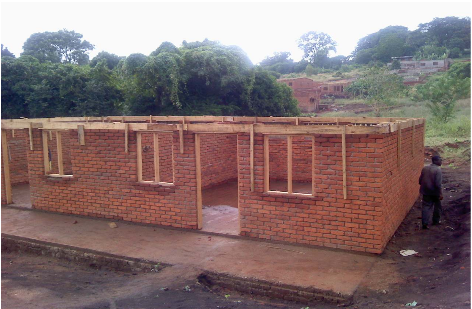
Pic.6: Womens Shelter-Front/Side View
